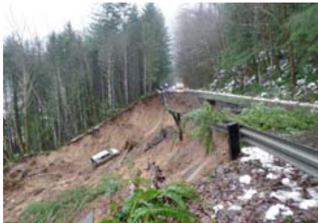
January 2012 landslide on USFS Road 15 to the Andrews Forest. Photo by Mark Schulze.
