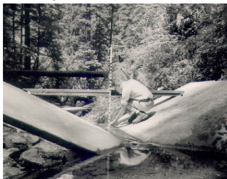
(Above) Jerry Franklin measures water depth at the weir in Watershed 1 at the Andrews Forest in 1957. Photo by Jack Rothacker. (Right) A tower supports instruments to sample carbon flux in the air stream flowing out of the Watershed 1.
