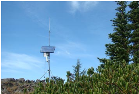
Wireless communications tower being tested at the Andrews Forest. Photo by Adam Kennedy.
