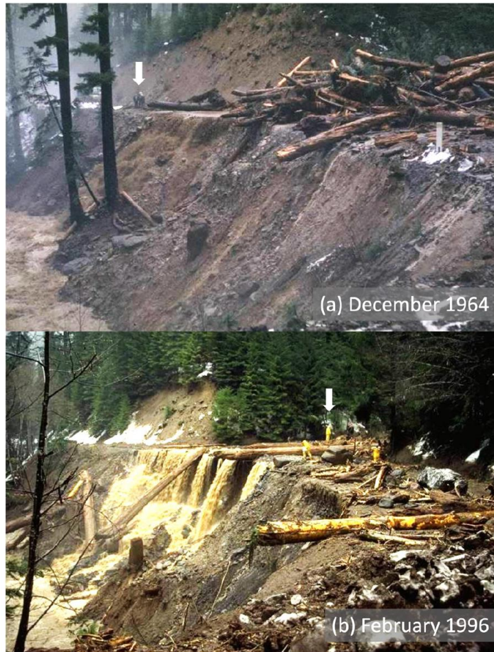
Figure 5 in Goodman et al. 2023. Photographs of debris flow deposits on the road passing by the mouth of the Watershed 3 stream (entering from the upper right) where it reaches Lookout Creek (lower left) (see location in Figure 4). (a) Pile of large wood delivered by the third pulse of multiple debris flows from watershed 3 on the night of 22–23 December 1964. Two previous pulses occurred during the night and early morning of 21–22 December (Fredriksen, 1965). Thirty-two landslides moved an estimated 30 000 m 3 of sediment (300 m 3 /ha) in the watershed. Twenty-nine of the 32 landslides were adjacent to stream channels, and 93% of the material originated from roadrelated slides (Fredriksen, 1970). (b) Deposit from debris flows on the night of 6–7 February 1996 showing fewer very large wood pieces in 1996 compared to 1964. Note human figures for scale indicated by white arrows. Photo credits: 1964, Dick Fredriksen; 1996, Al Levno.
