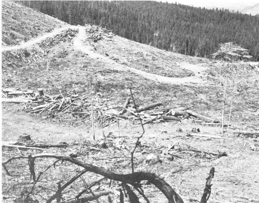
Figure 8. Severe soil compaction on forest roads, landings, skid trails, and other areas disturbed during logging can cause overland flow. As a result, size of peak flows of streams draining logged watersheds may be increased.
