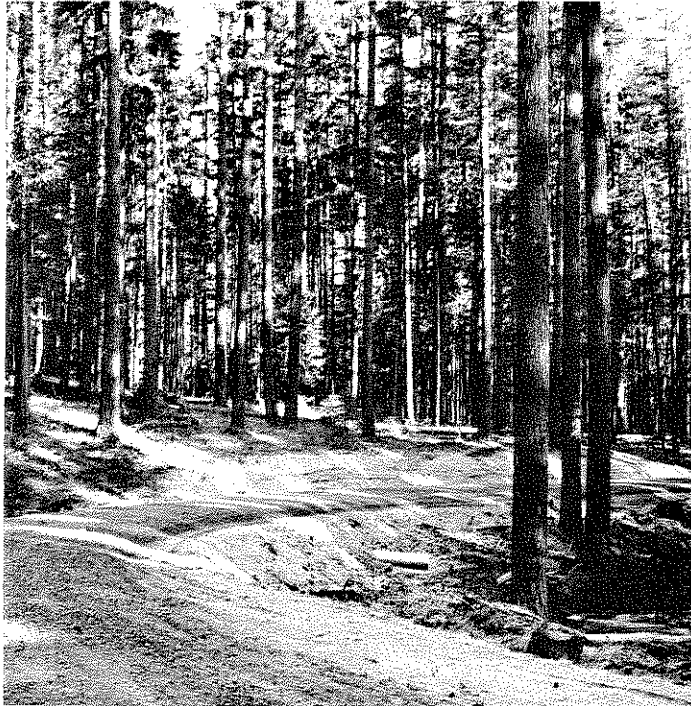
Figure 4.--Newly constructed road with mulched cutbanks and fill slopes in CC-2.
