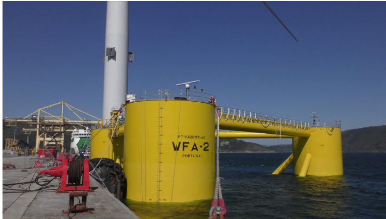
Figure 10. Floating offshore wind turbines at assembly ports. Top: Floating wind turbine (9.5 MW) for Scotland’s Kincardine Offshore Wind project at a port in The Netherlands. Bottom: Floating platform for an 8.4 MW Floating wind turbine for Portugal’s WindFloat Atlantic project along a quay in Spain (for scale, note the figure in red coveralls at the top right side of the floating platform). Photographs courtesy of Principle Power.
