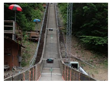
This view looks up the flume from inside the unfilled pond, the walls of which were constructed of concrete divider blocks and sealed with commercial-grade, expandable orange
