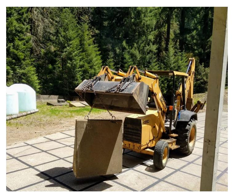
Lifting roughly half-ton concrete blocks to assemble a makeshift "pond" at the base of the flume required heavy-duty chains, a temperamental tractor, and a skilled operator. Credit: USGS
