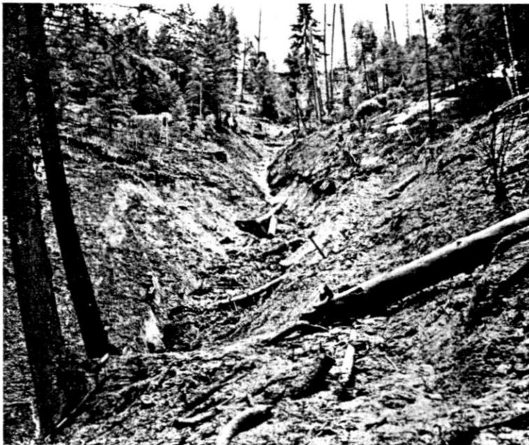
Figure 3-c. Debris torrent developed in an intermittent stream channel along the South Fork of the Salmon River in Idaho. Initial failure occurred in road fill near the ridgetop.
