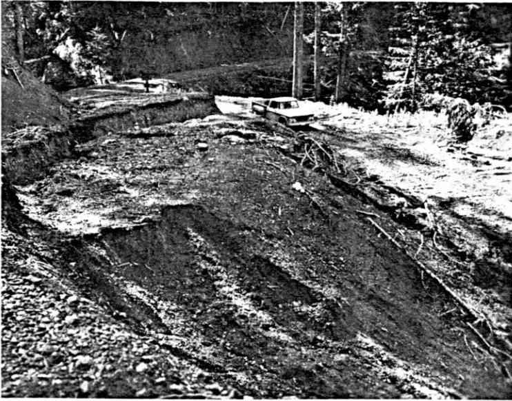
Figure 6. Examples of mass soil movements resulting from failure along a road right-of-way.
