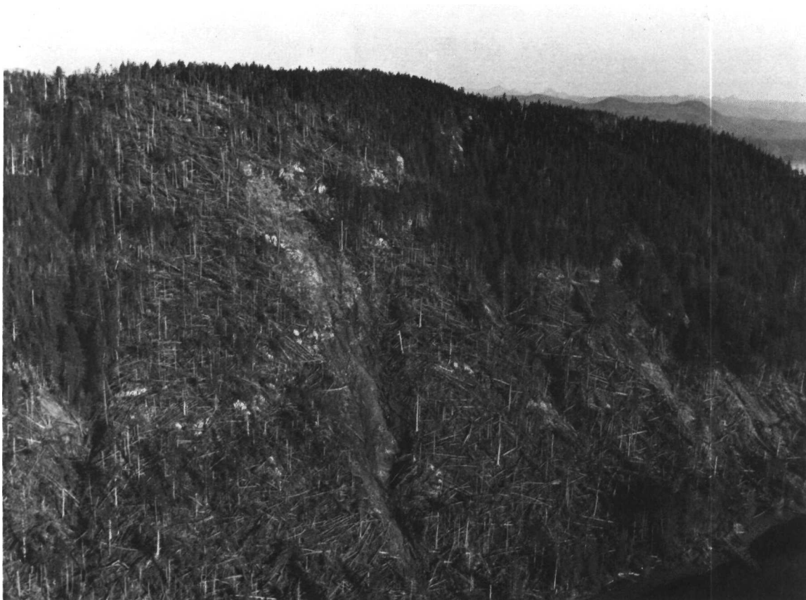
Figure 8.—One storm in November 1968 blew down millions of board feet in stands as shown here. Also note the landslide in the center of the picture.
