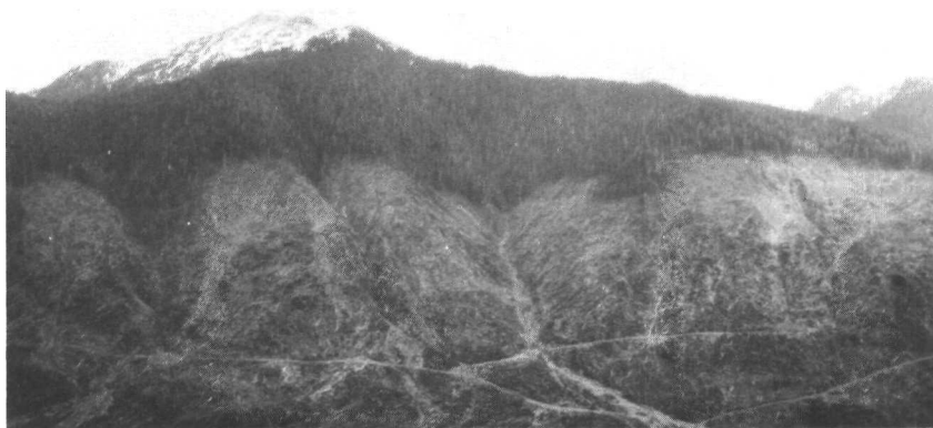
Figure 3.--Debris torrents developed in deep, V-notch side drainages to Maybeso Creek, Prince of Wales Island. All three developed initially above the cutting boundary, probably due to failure of a natural debris dam.
