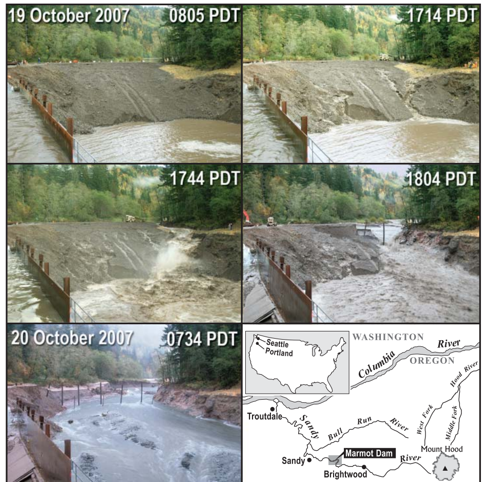
Fig. 1. Location of Sandy River, Marmot Dam and time-lapse images of the temporary earthen dam. The first image, at 0805 Pacific daylight time (PDT), was taken before the pumps dewatering the earthen dam were removed. Shortly after the pumps were shut off, water began seeping through the dam, gradually triggering small mass failures. Once all of the pumps were removed, crews carved a small notch in the dam crest and released the impounded water. Note the seepage and mass failures on the dam's downstream face evident by 1714 PDT; the channel and small knickpoints that developed as water overtopped the dam after it was notched, and the migrating headcut in the reservoir following breaching. By the following morning, the earthen dam and a substantial volume of stored sediment had been removed. Exposed well casings are about 10 meters tall. Note people for scale in some images. Data shown in Figure 2 were collected at U.S. Geological Survey gauging stations near Brightwood, Ore., and 450 meters downstream of Marmot Dam. Portland, Ore., is located 20 kilometers west of the Sandy River/Columbia River confluence.
