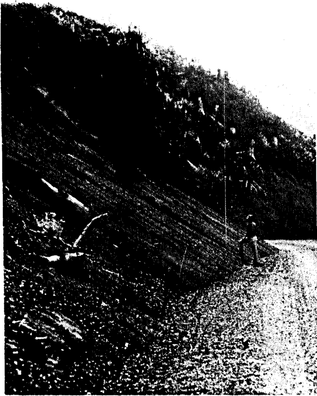
Fig. 5. Dry ravel from a road cut in western Washington.
