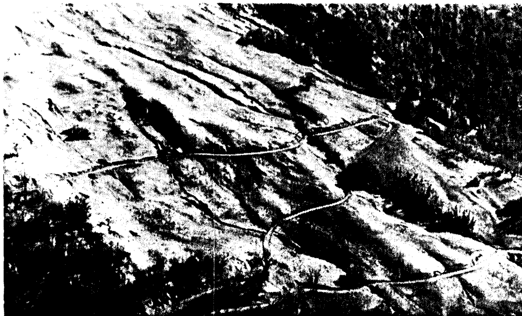
Fig. 4. A watershed slope in the Coast Range of northern California undergoing massive creep and slumping. Note deep gullies within intermittent drainage channels and below road cross-drains. The slope is undergoing creep, as indicated by the hummocky nature of the surface, with local slumps occurring below spring outlets and above road cuts. Numerous springs at the surface suggest that the entire soil mass is well lubricated with water, probably the chief mobilizing factor.
