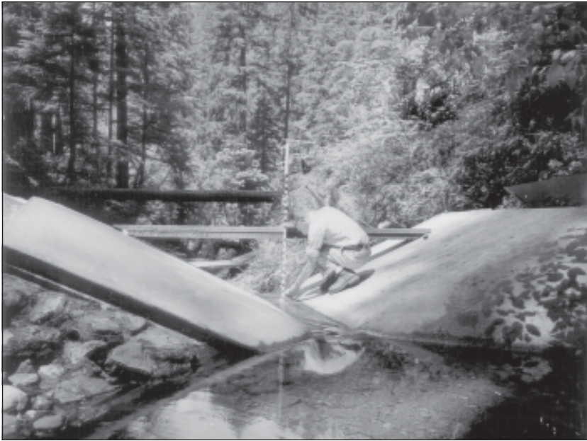
Figure 14—Jerry Franklin, shown here measuring streamflow with a velocity head rod at the weir, experimental Watershed 1 gaging station in July 1957, was one of Rothacher’s earliest associates at the H.J. Andrews Experimental Forest.
