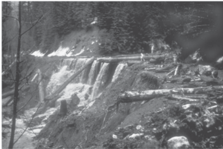
Andrews Forest Watershed 3 stream flowing over debris flow deposits and road into Lookout Creek (lower left) during the February 1996 flood. Debris flows originating from roads and forest areas periodically disturb small streams. Figures in background are Fred Swanson, Gordon Grant, and others. Photo by Al Levno, USDA Forest Service.
