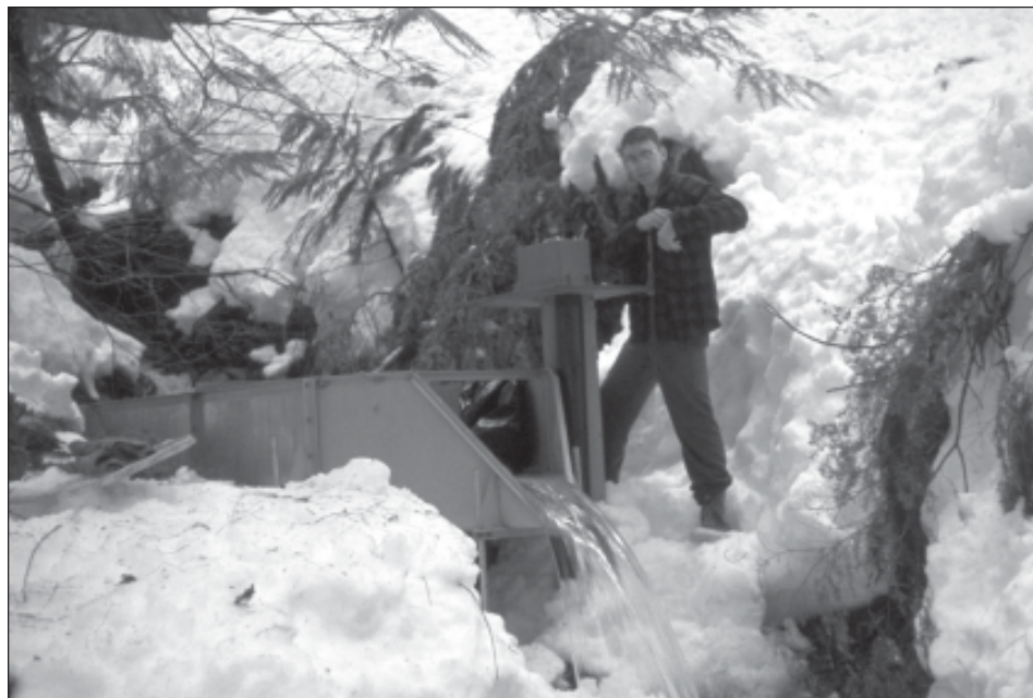
Figure 24—Watershed (WS) 7 was the first watershed to receive a gaging station in the “Hi-15,” three experimental watershed set, which includes WS 6 (32.1 acres), WS 7 (38.1 acres), and WS 8 (52.9 acres). These watersheds are located on a south aspect at around 3,280 feet elevation. They contain 130-year-old Douglas-fir. An H-flume was installed at WS 7 in 1963, with a FW-1 recorder with a 7-day chart that continuously recorded water levels. Technicians built shelters over these H-flume installations shortly after they were installed to protect them from snow “bombing” off overhanging trees during winter. Here, Al Levno checks the installation during the first winter after construction in 1964.
