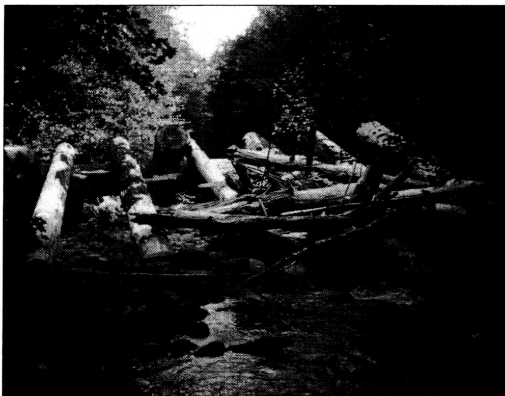
Quartz Creek trash rack.
