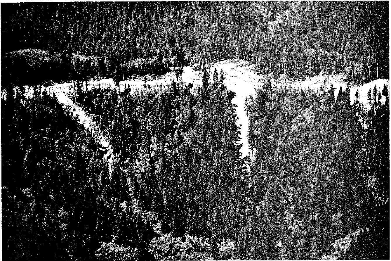
FIGURE 18. Road slumps and slides from a logging road in the Deer Creek watershed.
