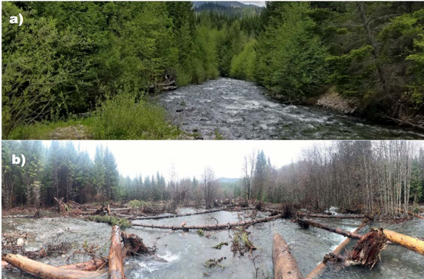
Figure 2.2: Stage 0 restoration project on Lower Staley Creek (a) before restoration in Summer 2017, and (b) a few months after restoration in Fall 2017. Photos courtesy of Matt Helstab (USFS) and Johan Hogervorst (USFS), used with permission.
