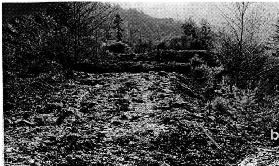
Figure 2.4. An example of the least intensive road rehabilitation technique. a) Abandoned logging road before treatment. b) The road surface is decompacted, and ditches are constructed perpendicular to the road alignment to drain the road. The road bench and road fill remain in place.
