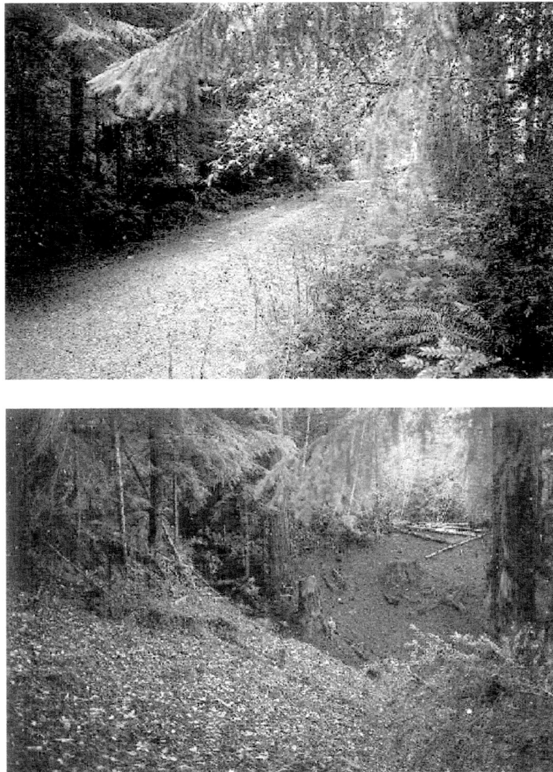
Figure 2.5: An example of the most intensive road rehabilitation technique. a) Abandoned logging road before treatment. b) The road bench is obliterated and the hillslope recontoured (total outslipping of the road bench, and total excavation of the stream channel). Note person for scale next to a stump that was exhumed during channel excavation.
