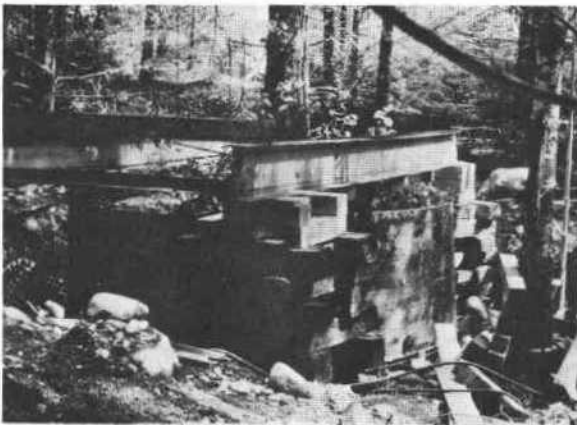
Figure 2. Completed inner container with soil and tree shown raised 90 cm for installation of the hydraulic transducer.
