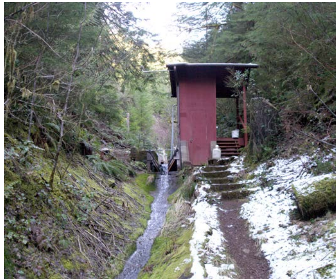
Figure II.B.7.2. Gauging house and channel below flume at Watershed 10 gauging station.
